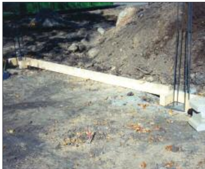
Figure 1: AB Fence Pile Layout Jig
