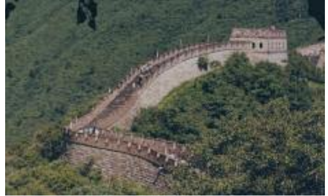
The Great Wall of China, dating back some 2,200 years, was built as a double sided retaining wall. The soil between the two walls was a mixture of clay and gravel reinforced with Tamarisk branches. Allan Block retaining walls employ "old technology with new materials."
