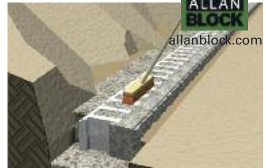
Sweep to remove excess materials for proper placement of next course.
