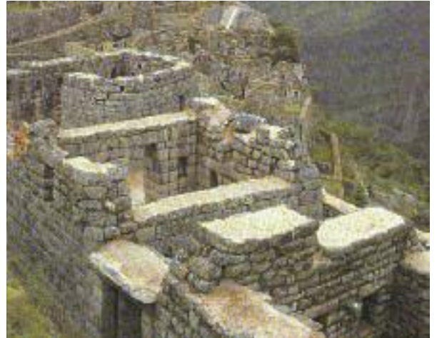
Mortarless construction has been used for centuries.
