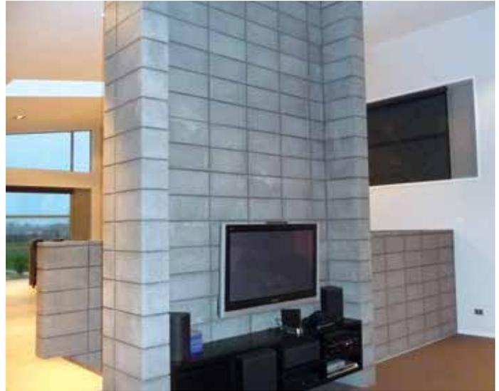
Chipping should be limited to 5% of a consignment containing less than 12.5mm in any dimension and any cracking to be less than 0.5mm in width and less than 25% of the nominal height of the unit.
