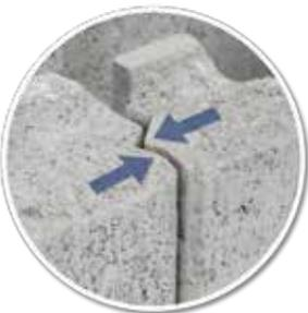
Interlocking tongue and groove joints
