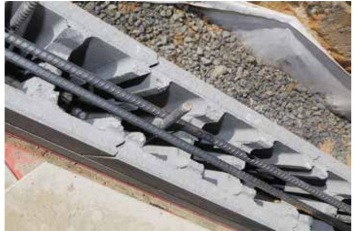
\*4 hour fire rating for Versaloc® 200mm and 300mm series. 2 hour fire rating for Versaloc® 150mm series.
