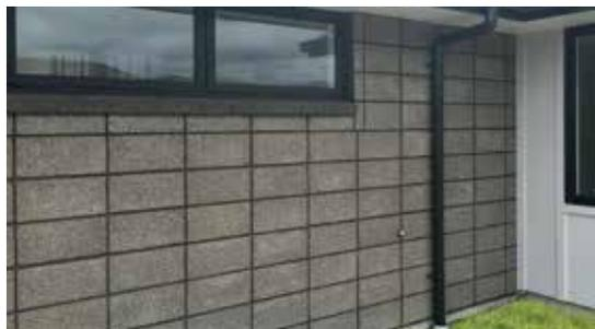
Stack Bond is outside the scope of NZS 3604 & NZS 4229 and requires specific design.
