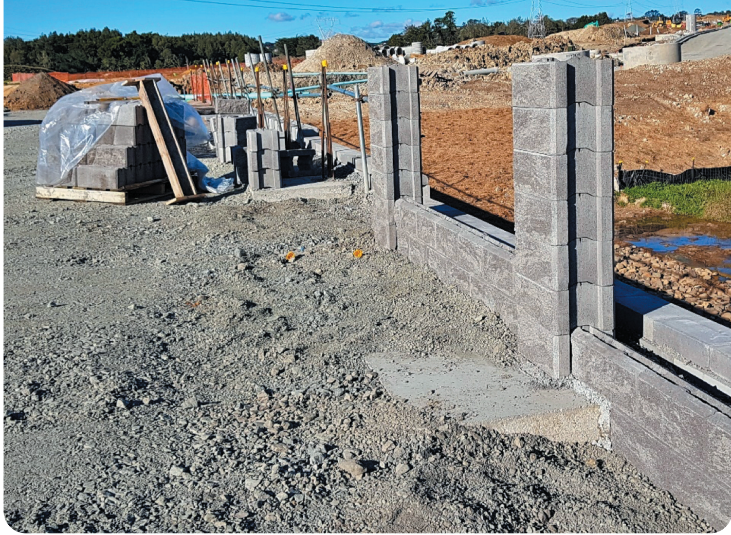
Figure 3: AB® Fence with a cantilevered footing
