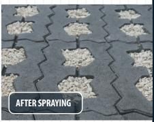
Keep traffic, both pedestrian and vehicular, off the sprayed surface to avoid marking or dirt sticking the drying solution. A finger touch test will indicate when the solution has dried.
